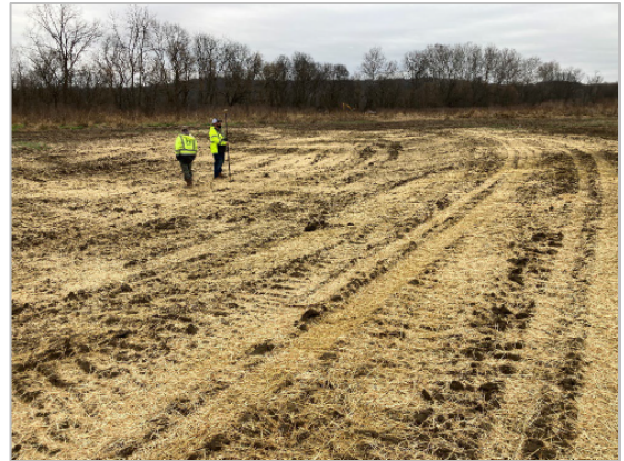
Spot checking grade of middle wetland pool
